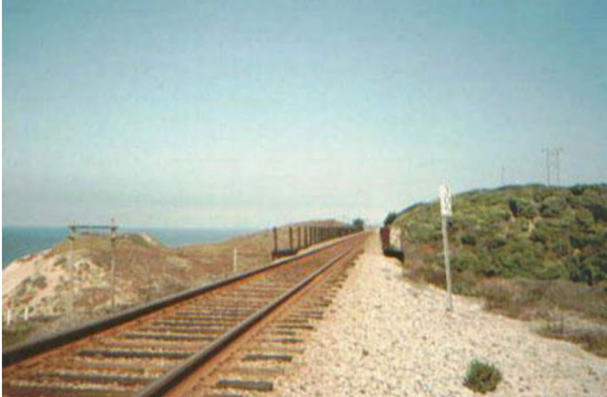
Figure 3. Honda Section House location along the Southern Pacific Railroad on Vandenberg Air Force Base.
