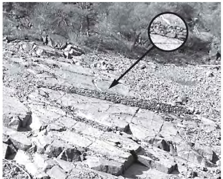
Figure 3: Running across the center of this photo, a surviving segment of the Big Bend Mule Trail is anchored to what is now the exposed bedrock of the Lake Oroville fluctuation zone. Inset enlargement shows detail of the carefully built stacked-rock retaining wall supporting the trail. The wall is roughly five feet tall at its highest point (Anthropological Studies Center photo).
