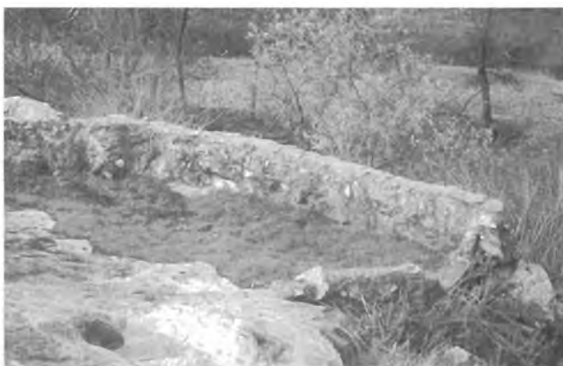
Figure 18. Stone and mud-mortared catch-basin from the late 18 th or early 19 th century.
