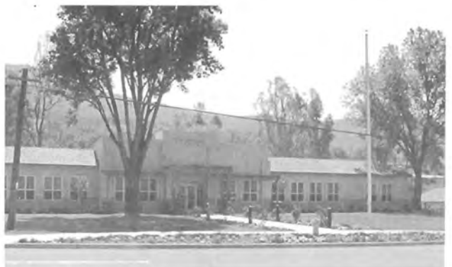
Figure 12. The San Pasqual Academy after renovation in 2001.
