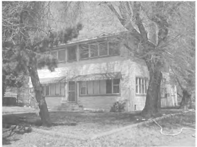
Figure 2. The Olds residence, oblique view.
