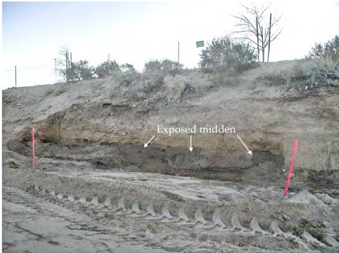
Figure 1. Midden exposed during construction (Love 2015a:6)
